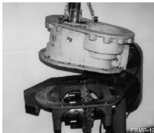
Picture 20: Installing of the spur gear housing
